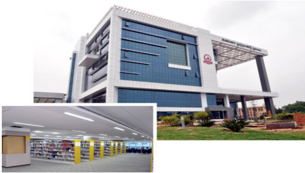
Fig. 1. Anna Centenary Library, Chennai ( https://www.annacentenarylibrary.org/ )
