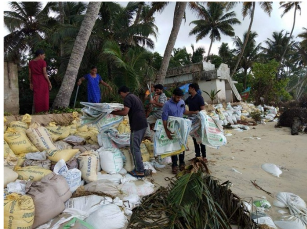
Picture 1: Temporary Sea Wall Construction by NSS Volunteers
