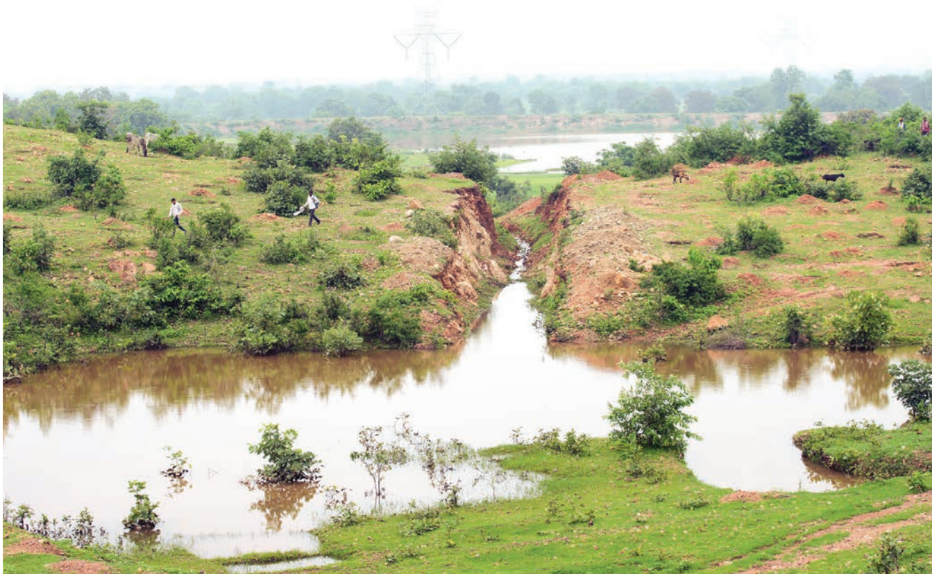
Women of Agrautha village in Chhatarpur cut through a hill to devise a channel that directs runoff during monsoon to a pond
