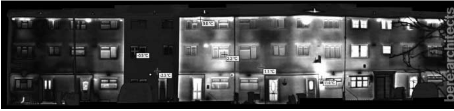
Figure 21.6. Thermal Image of Passfield Drive, East London, 8.30 A.M. on January 31, 2012. Light areas show high heat loss across the terrace. Dark shows the positive effect of a Passivhaus retrofit. Courtesy of bere:architects.
